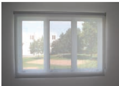
View from inside through a double-clear low-e window with an interior reflective roller.
