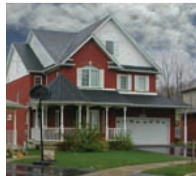
Tucking the garage below habitable space can be an attractive and effective solution.
