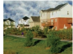
Turning a back lane from gray to green offers a traffic-free path for residents.
