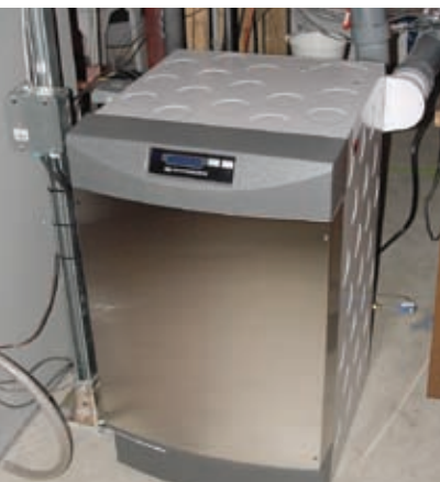
The Stirling engine installed beside the furnace provided an initial stage of heating and electricity to the house.
