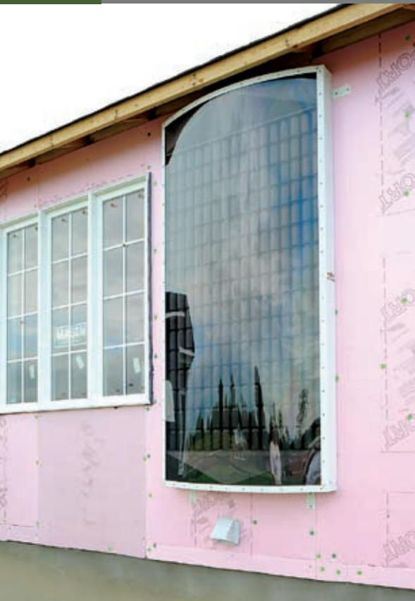
One example of energy savings through renewable energy is found in a solar heating unit manufactured with recycled content.
