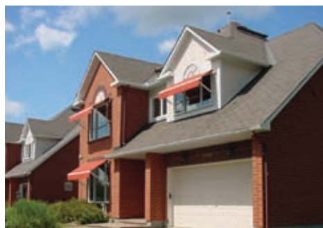
The awnings are expected to result in a seasonal saving of 401 kWh or 15 per cent.
