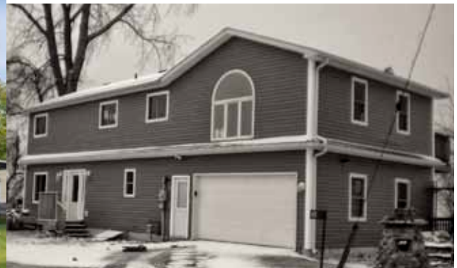
The exterior façade is now comprised of custom painted Egyptian Blue board and batten siding accented with contrasting white features.
