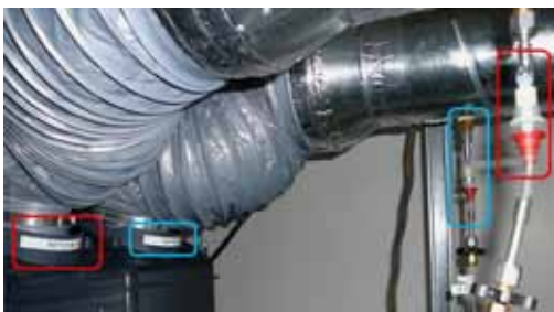
Figure 2: Air sampling for determining supply (blue) and return (red) air quality
