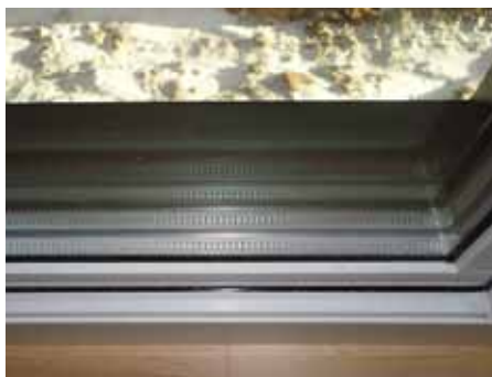
Triple pane windows reduce noise transmission and add increased insulation with an added pane of Low E Argon Gas.
