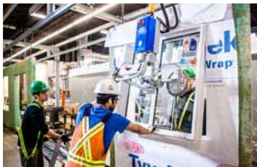
ACQBUILT employees ensure windows are installed with precision and accuracy.
