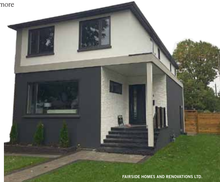
FAIRSIDE HOMES AND RENOVATIONS LTD.
